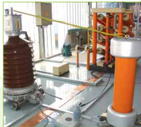
Measurement of leakage current
